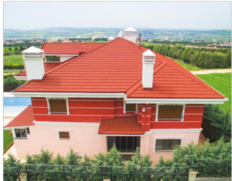
Starbond's Metal Tiles are made of % 55 Aluminum-Zinc (ALUZINC®) alloy coated sheet steel that is knowns as GALVALUME® .This product is water-resistant and corrosion-resistant. It has a structure that allows the reflectivity of the heat and support Climatic insulation in buildings (cold or hot) and shows the effect of shield . The characteristic of being light, it does not put load buildings, cut and bent, transport and installation is easy
